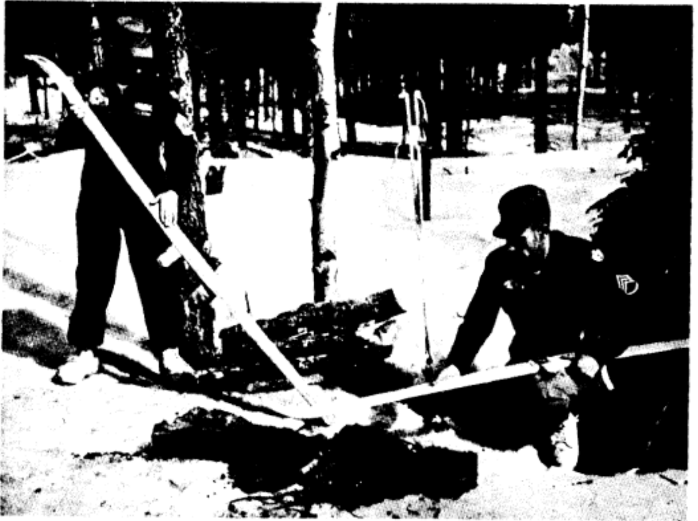
Figure 4-6. Heating skis over an open flame.
